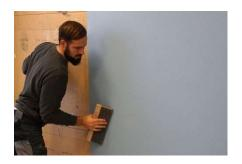
During the installation and the bonding of the adhesive, noraplan® wall coverings have to be protected against extreme heat or temperature fluctuations, e. g. as a result of direct sunlight or in rooms where glazed elements reach down to the floor.
