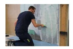
When the wall covering is embedded, it has to be ensured that its entire back is completely covered with adhesive. Position the edges of the wall covering without applying pressure. Under no circumstances should they be pressed or crushed. As the joints have to be sealed, the joint width must not exceed 0.3 mm.
