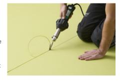
5. The processing temperature is 350-400° C (for noracare™ max. 300° C). Set the speed to approx. 2 linear metres/min. The operating speed and temperature can be regulated on most welding machines.
