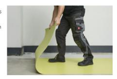
6. Cut and remove the protective paper of nora dryfix™ 750, leaving an approx. 10 cm length from the flooring. Fold this 10 cm length underneath the flooring that has been folded back. This is meant to keep dirt particles away from the adhesive layer.
