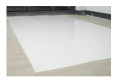
3. You can either trace-cut (using a ruler as a guide) or double-cut the seam between two nora dryfix™ 750 strips. Take care not to leave any gaps wider than 2 mm.
