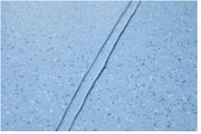
**6.** The surplus cold weld pressed to the sides can be removed after approx. 12 hours.
