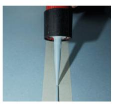
5. Immediately after application, the cold weld is pressed into the joint and smoothed with the big round shape of the nora® smoothing spatula.
