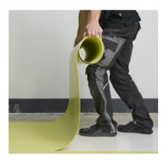
**5.** For sheet flooring, fold back half of its length; for tiles arranged in a row, work your way from the center and lift each tile up as required.
