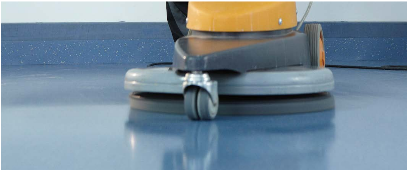
Finishing. Clean coverings first and then polish to a high gloss
